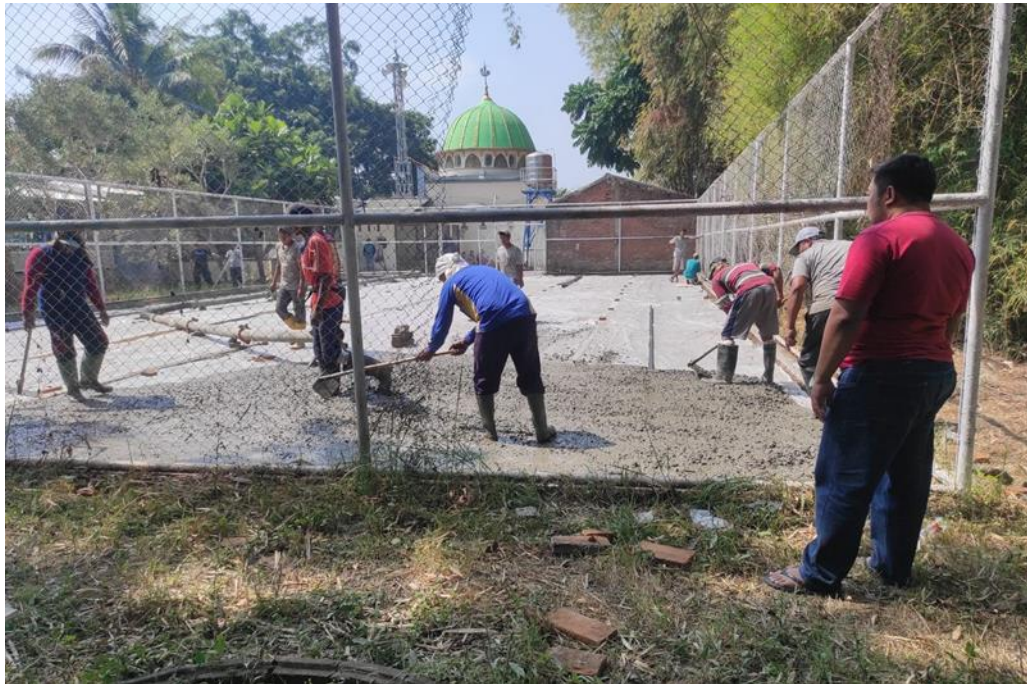
Figure 3: Cleaning and casting of the sports center.
